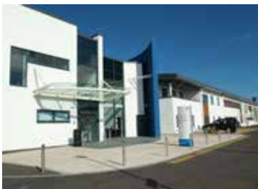
Crosshouse Maternity Hospital, UK
